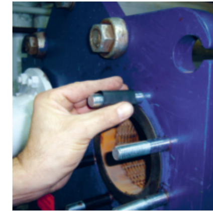
Shuffle the shrinking hose about the bolt
